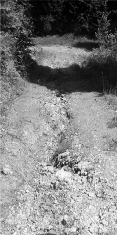
**Figure 1. The impact of the water to the non-existence road drainage system.**
